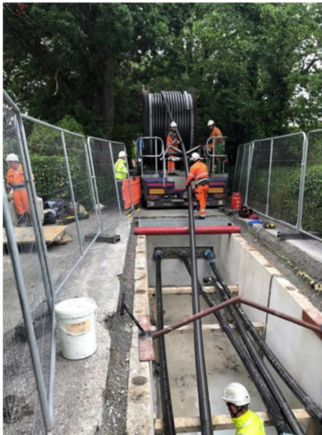
Figure 2-8: Typical Set-Up of HV Cable Pulling Procedure
