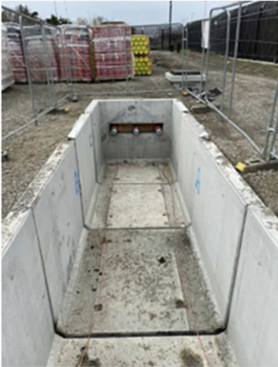
Figure 2-8: Typical Set-Up of HV Cable Pulling Procedure
